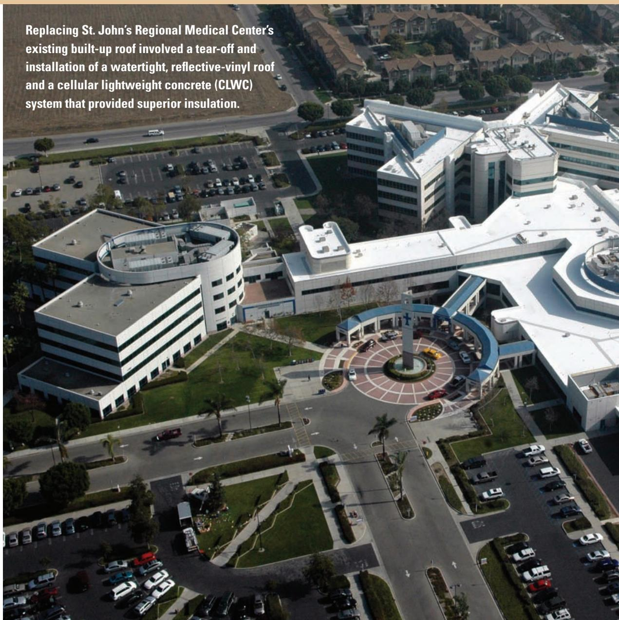
Replacing St. John's Regional Medical Center's existing built-up roof involved a tear-off and installation of a watertight, reflective-vinyl roof and a cellular lightweight concrete (CLWC) system that provided superior insulation.
