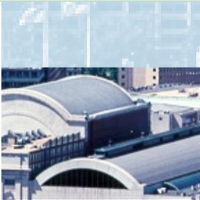
**Watertight, UL-listed vinyl membrane was selected to protect the structural and historical integrity of Washington, D.C.'s Union Station. Rehabilitation of the arching barrel roof without ruining the priceless suspended plaster ceiling underneath or old cement falling on the shoppers and travelers below were key requirements.**
