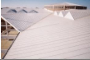
**A failing low-pitch shingle roof system on three elementary schools joined by a central rotunda in Plano, Texas, was replaced with the leak-tight security of hot-air-welded vinyl. The light gray reflective membrane formed tight seals around the rotunda's complex curvatures, and rib-like extruded profiles were adhered to replicate the appearance of standing seam metal.**
