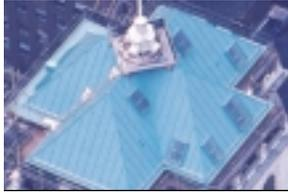
**Restoring the original, cosmetically critical roof of Times Square's Candler Building called for a highly weather- and pollution-resistant material that could simulate a batten seam copper roof and offer a long service life. A custom turquoise vinyl membrane provides both the aesthetics and the performance the project demanded.**
